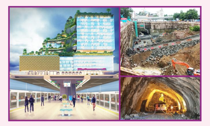
Swargate Multi Modal Transportation Hub (MMHH) excavation comprises of Underground Metro station with multi levels of commercial development above it and MMTH building consisting of 5 levels of underground parking, concourse and upper concourse levels. The total depth of excavation is enormous 28 m approximately.
